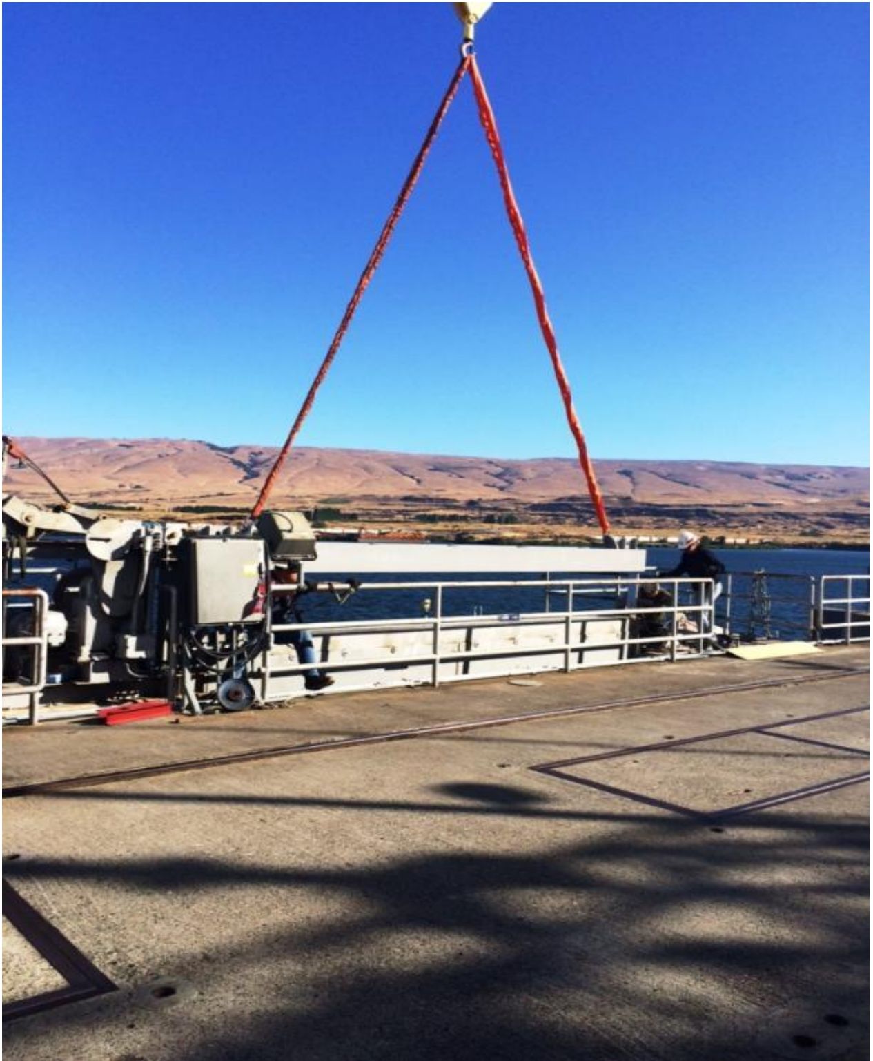
Ice/Trash sluiceway skimmer gate 1-3 refurbished and installed; used for juvenile passage.
